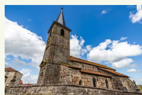
Fortified church Saint-Brice (Dombrot-le-Sec) - D2
